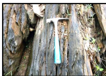
Fig 14. Vertical jointed nature of slate at near Kadaik Dam. (Loc. N16°44'28.1" E97°28'6.6", Facing 53°)
