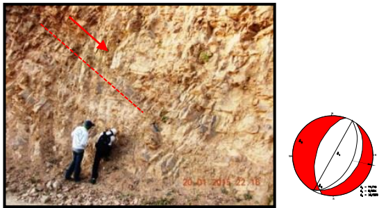
Figure (12). NW-SE striking normal fault on the siltstone unit of the Loi-an Group (20° 24' 58.9"N, 96° 38' 26.9"E) Photo Facing – 15°
