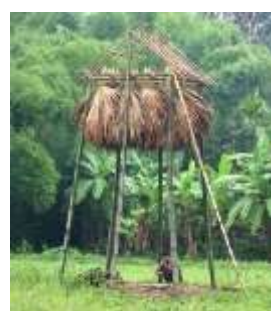
(C) Construction of roof
