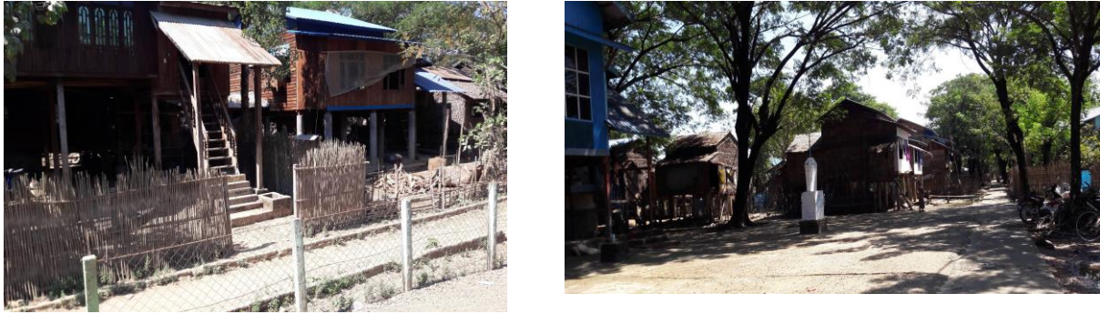
Figure (10). Photos showing the present house style in Thabaung Township. People in flood-prone villages build their homes upon a higher platform. If they cannot afford to build a higher floor, they have to relocate their houses to safer areas (Photo ©Khin Kay Khaing 2017)
