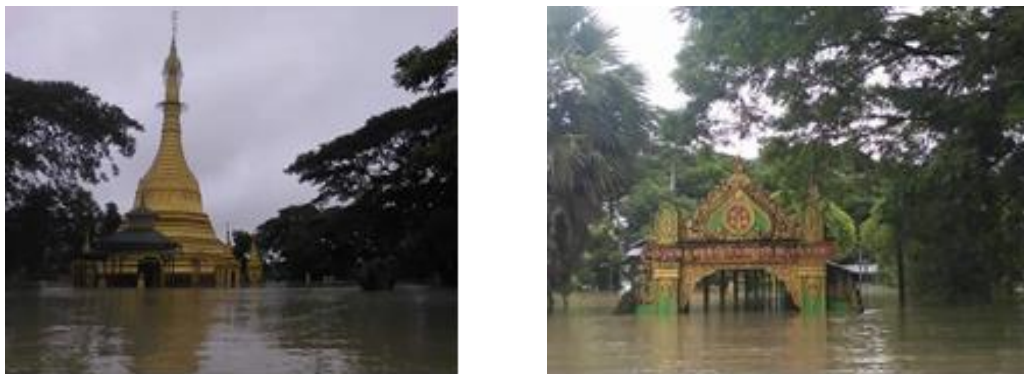
Figure (9). Pagoda and monastery in Htanzinhla Village, Thabaung in the 2016 flooding period (Photo ©Administrative Department of Thabaung Township)
